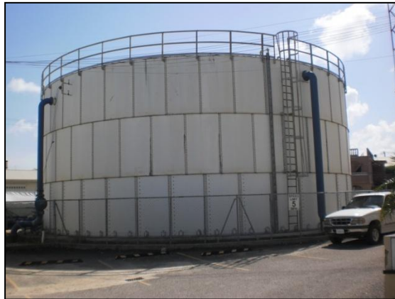
Southside Reservoir - Belize City
