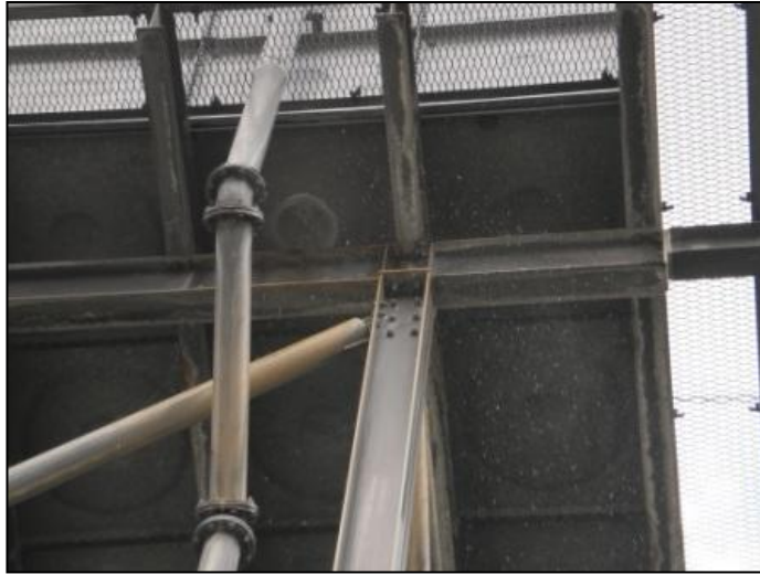
Leaking reservoir in Orange Walk
