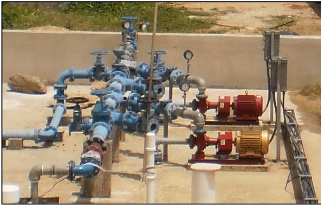
Pictures - New distribution motors/pumps, manifold, retaining wall and electrical control panel
